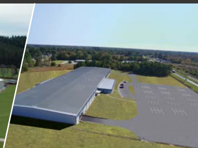
Plant Mullins/SC USA
