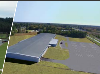
Plant Mullins/SC USA
