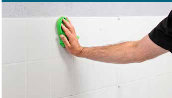
Clean old tiles and level out unevenness
